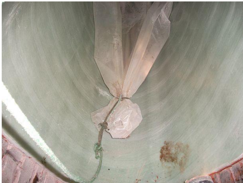
Figure 11: pulling of the inner film
